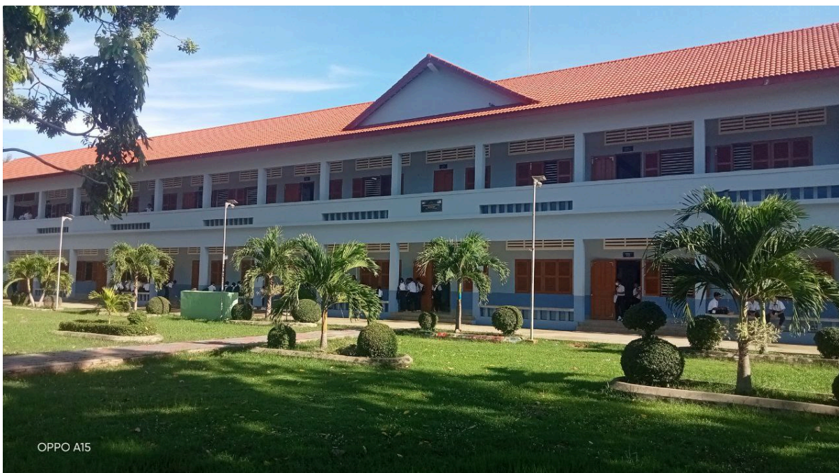
Physical Upgrading: Newly renovated classroom building at Preah Anduong HS in Prey Veng Province. ↗
