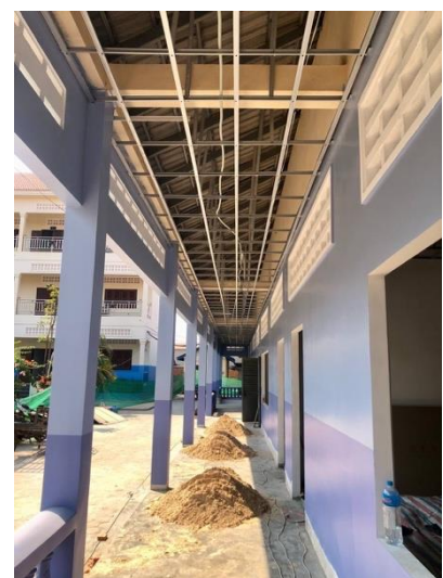
Renovations at a new NGS site in Siem Reap.
