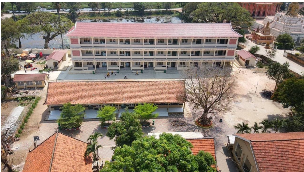
Large Investments in Primary School Infrastructure: A three-story building with 18 classrooms was recently completed at Akhea Mahasei PS in Kampong Speu Province.
